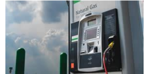
COMPRESSED NATURAL GAS
